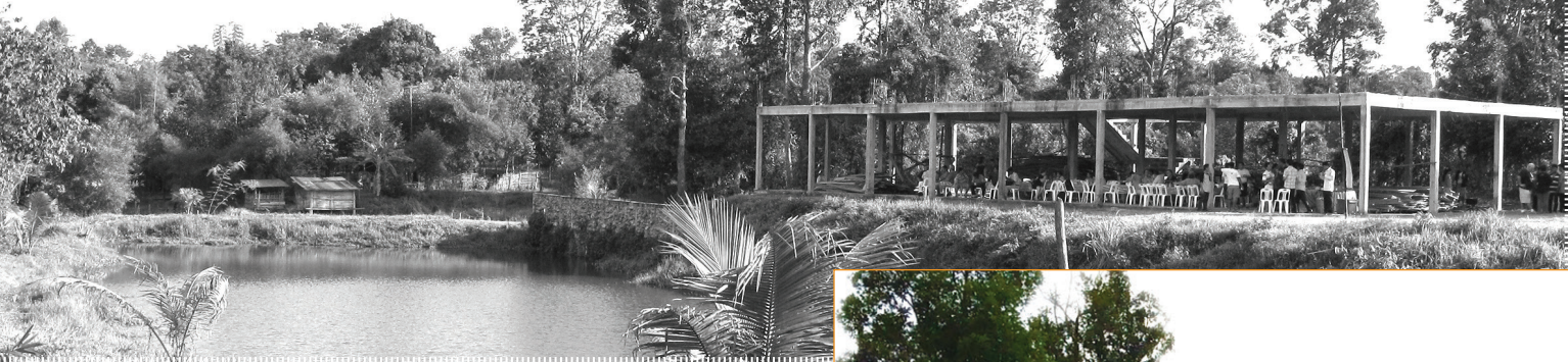
Acts College construction, start
