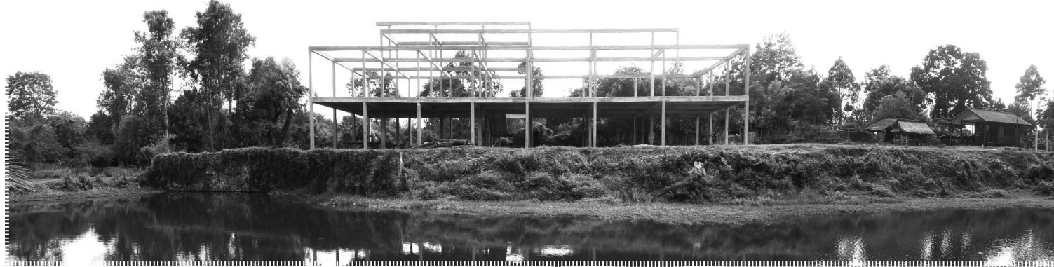
Acts College construction, continued
